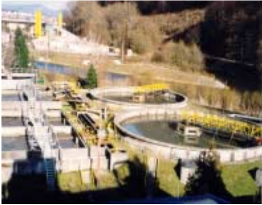
Waste Water Treatment Plant – Poland
